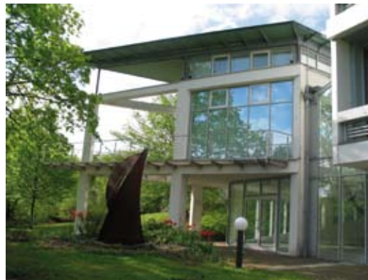
B-IT main building.
