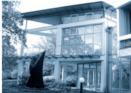
B-IT main building
