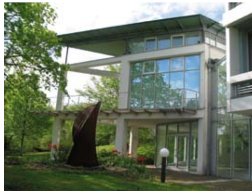
B-IT main building.
